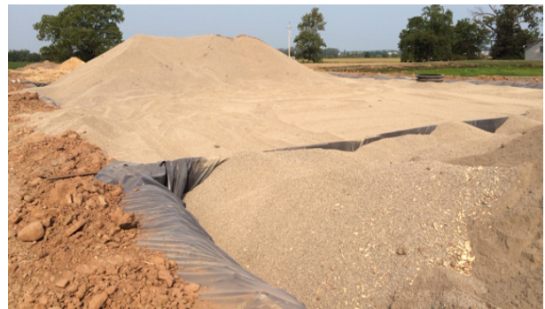
Figure 2: Mineral media cells under construction
