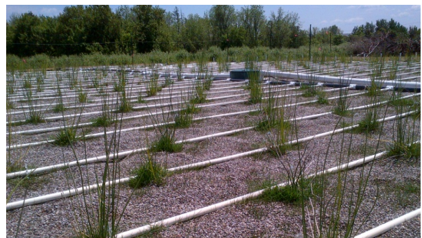
Figure 3: Newly planted vertical subsurface flow constructed wetland (Aqua Treatment Technologies)
